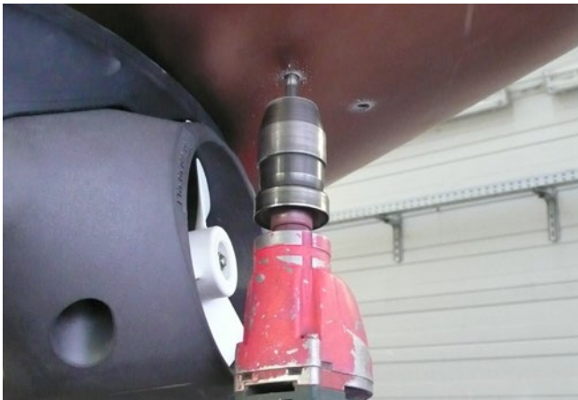
Fig. 19: mounting bolts drilling
